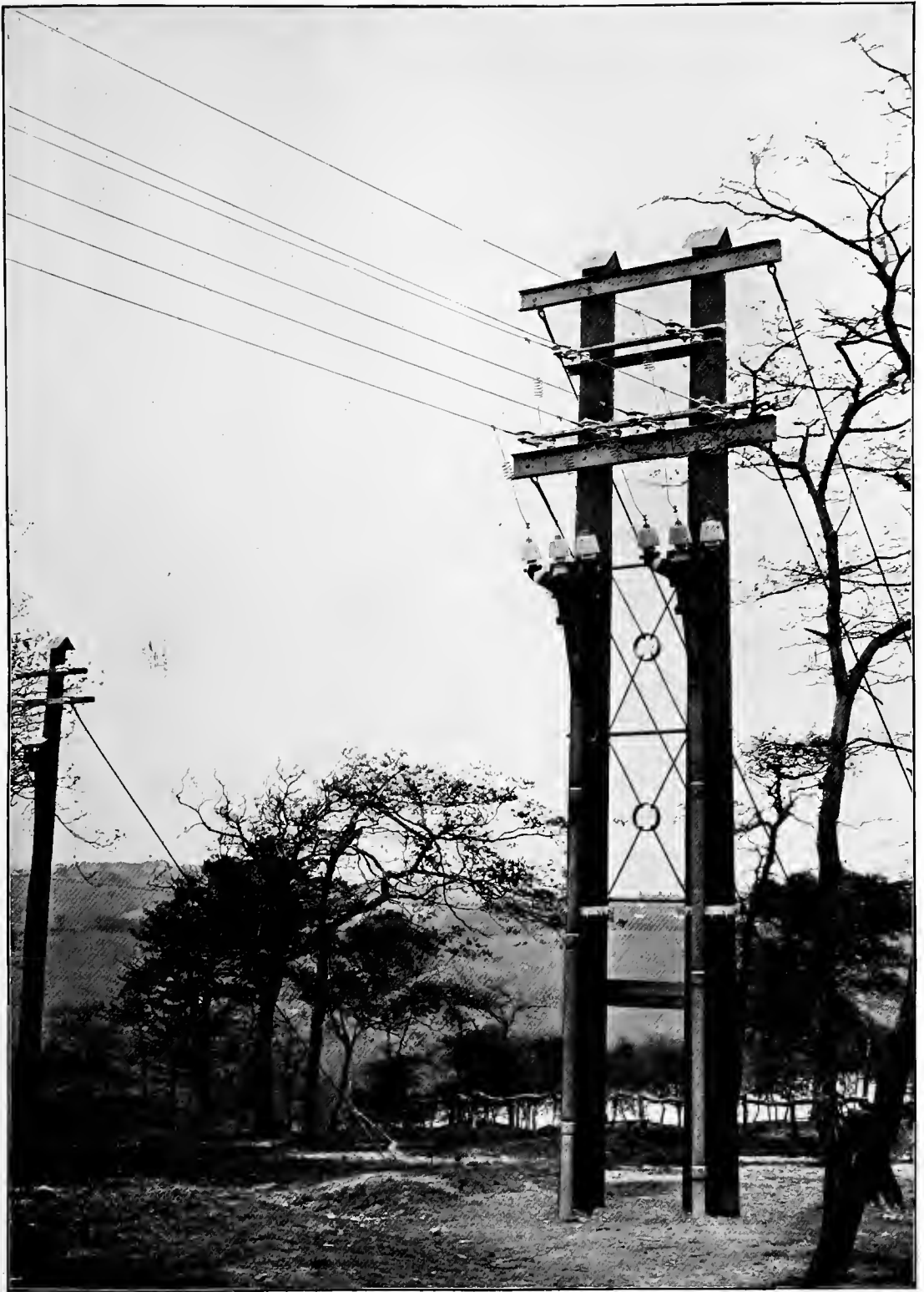
TERMINAL H POLE ON 10,000-VOLT TRANSMISSION LINE (WITH DIVIDING BOXES AND CHOKING COILS) (Callender's Cable and Construction Company, Ltd.)
